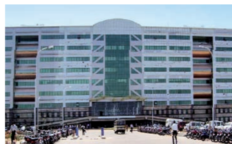
ETL Building, Indien
